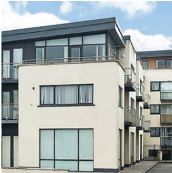
14 The Laurels 19 residential apartments, Tallaght, Dublin 24
